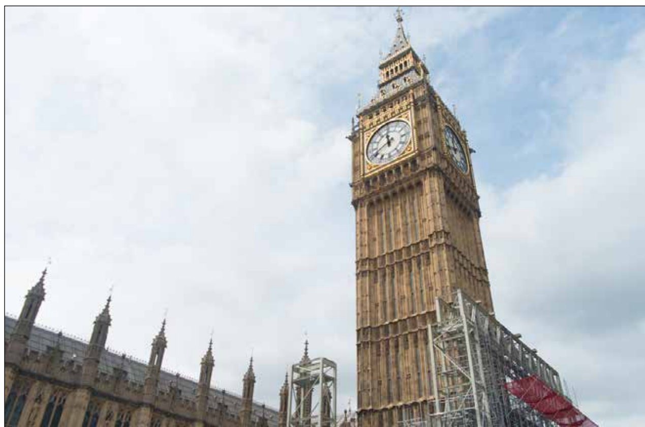
TIME FOR AN UPGRADE: Health and Safety regulations forbid Big Ben's bell to be rung during repairs
