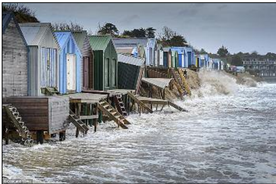
DAMAGE: Iconic beach huts that sell for more than £100,000 on the North Wales coastline have been devastated by the ferocious storms
