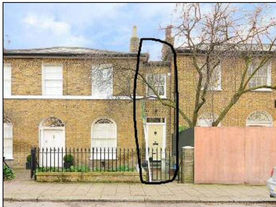
HOT MARKET: the five-foot wide house (ringed) covers just 538 square feet
