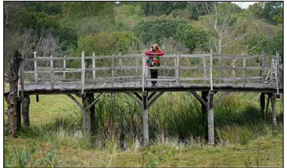
The original bridge, pictured, which featured in AA Milne's Winnie the Pooh books was replaced in 1999 and underwent restoration
