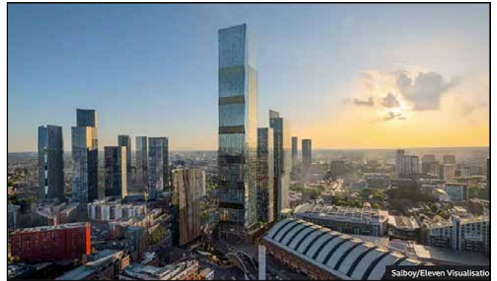
RISING SOON: the 76-storey building will be the UK's highest outside London
