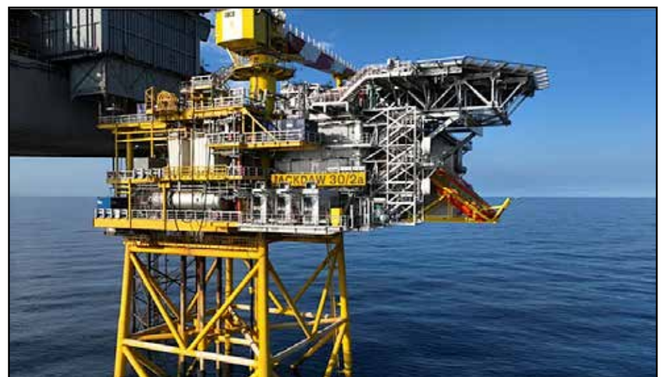
The Jackdaw rig will be situated due east of Aberdeen
